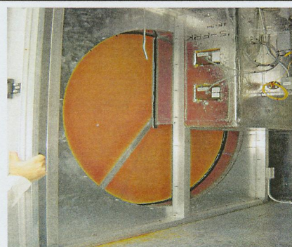
Desiccant Dehumidifier Package
