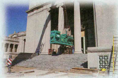
Chicago's Museum of Science and Industry now has an example of both — a 1.75 MW cogen gen-set that is the basis for both a scientific exhibit and an energy frugal power system. Photo courtesy of Cummins Power Generation.
